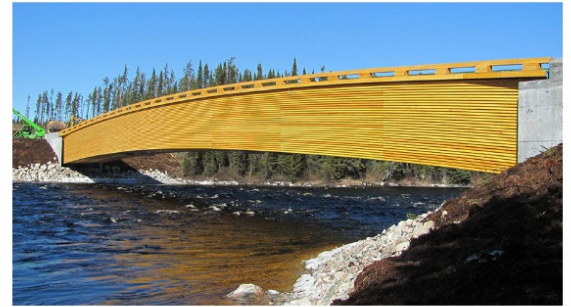
EWP bridge used for forestry operations in Maicasagi, Quebec. Bridge was designed and installed by Nordic Structures of Quebec.
